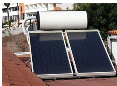
Fig. 12.3 Solar flat plate collector
